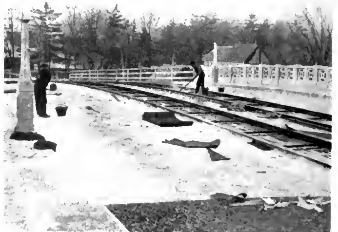
Deck view with waterproofing in progress.
